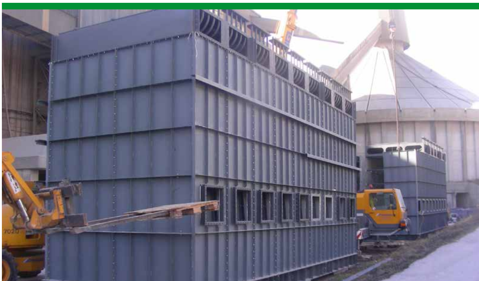
MENHOFER Rund-Schlauchfilter während der Montage. MENHOFER round-bag dust collector during the mounting.
