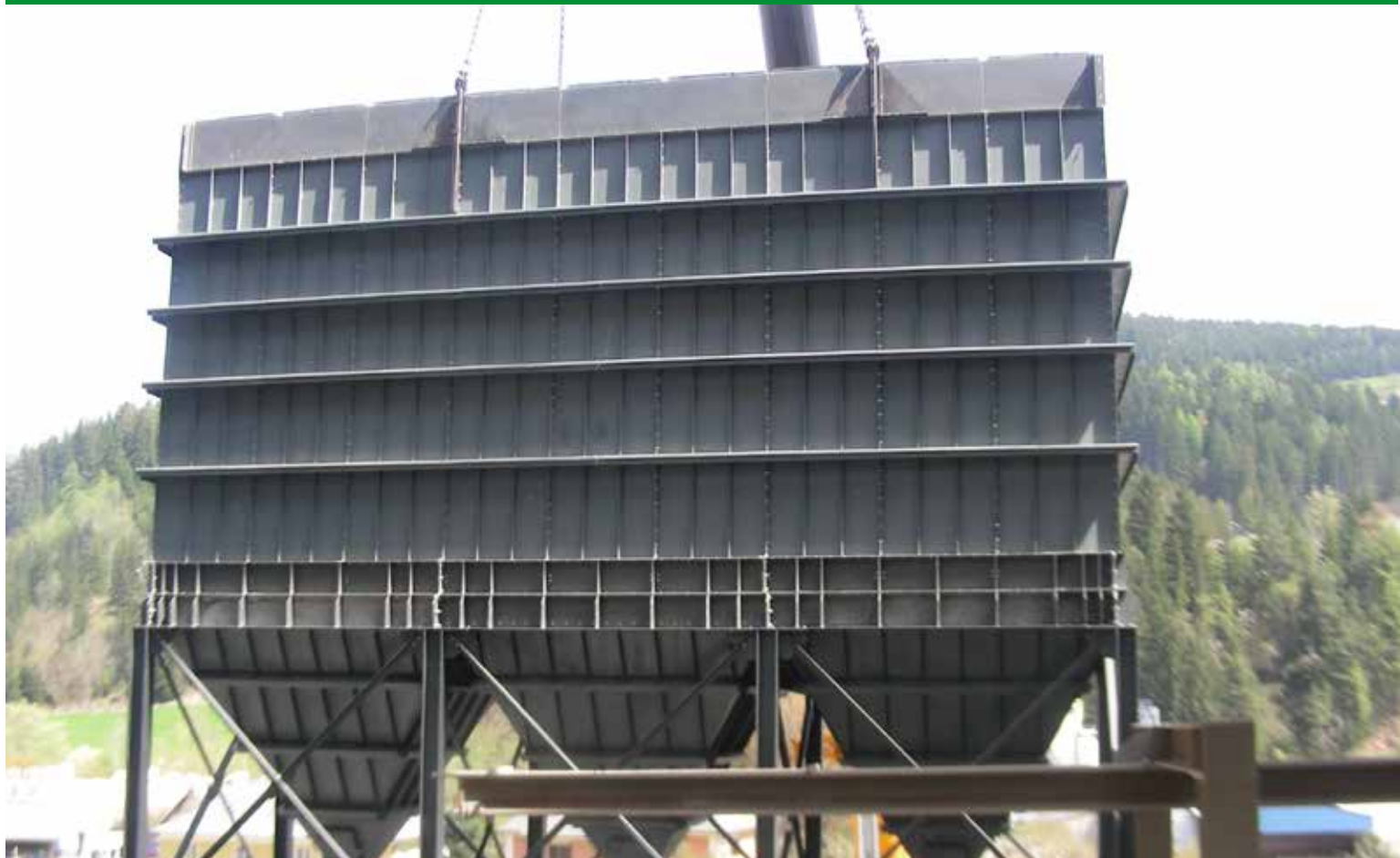
MENHOFER Rund-Schlauchfilter während der Montage. MENHOFER round-bag dust collector during the mounting.
