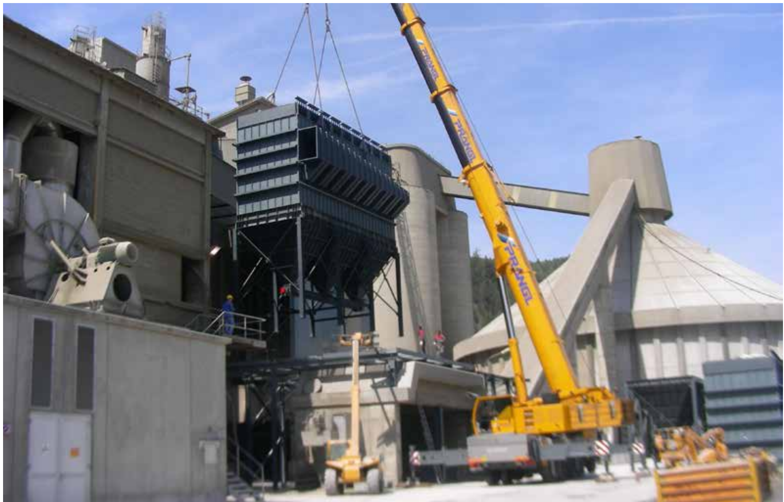
MENHOFER Rund-Schlauchfilter während der Montage. MENHOFER round-bag dust collector during the mounting.
