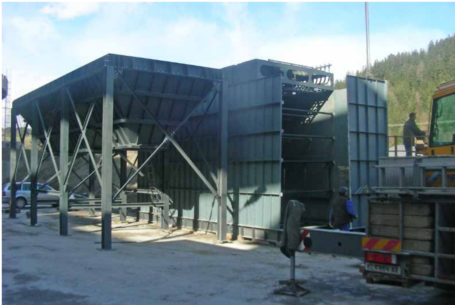
MENHOFER Rund-Schlauchfilter während der Montage. MENHOFER round-bag dust collector during the mounting.
